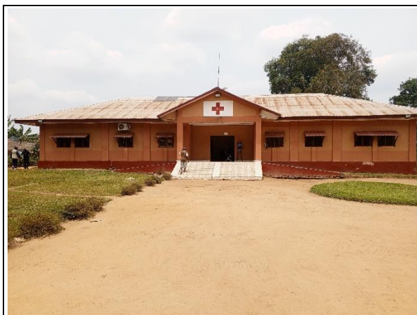
Photo 2. Centre Medical Moderne
